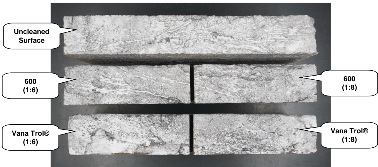
"Marana Textured" Solid Brick After Cleaning
